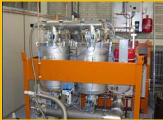
SOCOOL Trigeration system under construction
