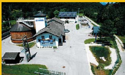
Sewage plant at the Hallstättersee (Source: www.rhv.at )
